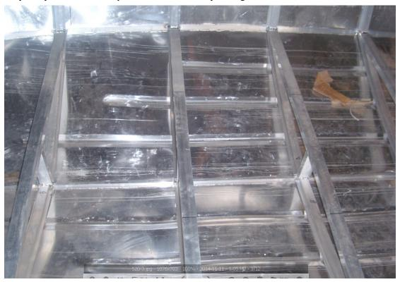
2.inside frame, all welded not fixed by bolt.
