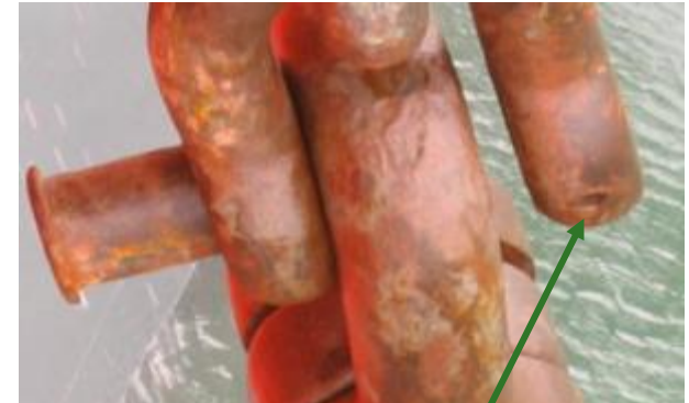
D-link bolt almost lost due to missing securing pin
