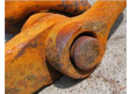
Worn out anchor shackle to be scrapped
