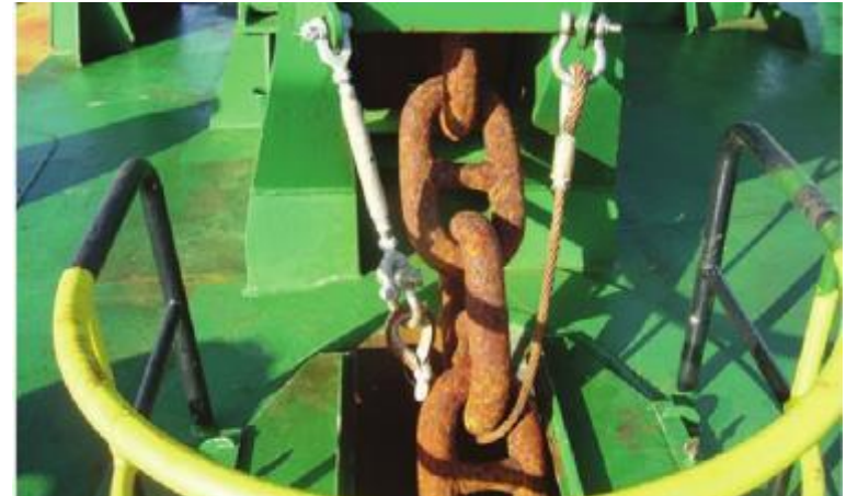
Securing of chain by turnbuckles (©OCIMF )
