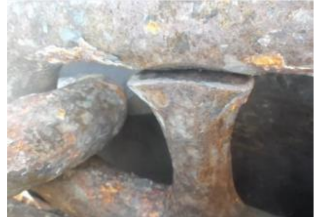
Stud with excessive gap
