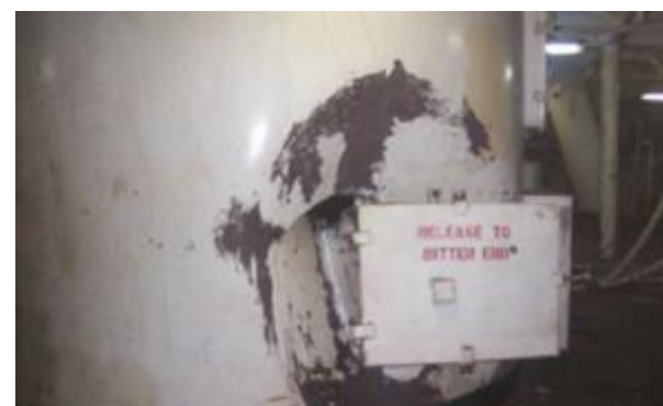
Anchor and chain lost due to windlass failure – damage to the chain locker in way of bitter end release
