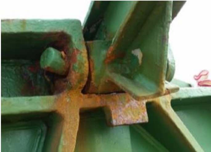
Chain stopper hinge pin severely deformed
