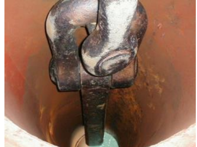
Anchor shank broken
