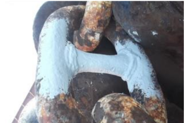
Un-authorized welding of stud
